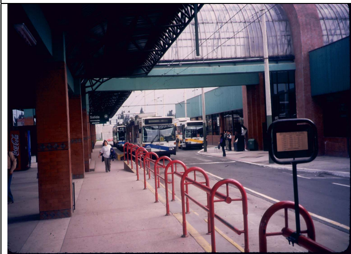
Photo 16 – Trolleybus Transfer Station/Terminal
