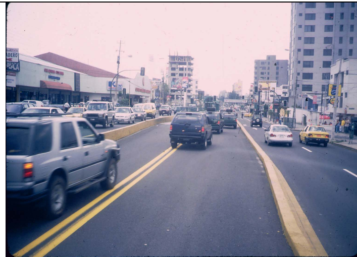
Photo 41 – Ecovía Exclusive Central Busway
