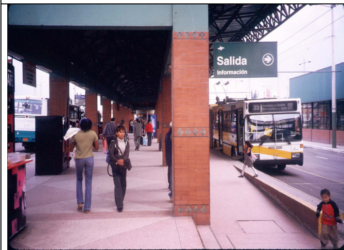
Photo 17 – Trolleybus Transfer Station/Terminal
