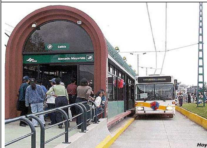
Photo 11 –Second Stage Busway - Bus Stop Platform (Trolleybus)
