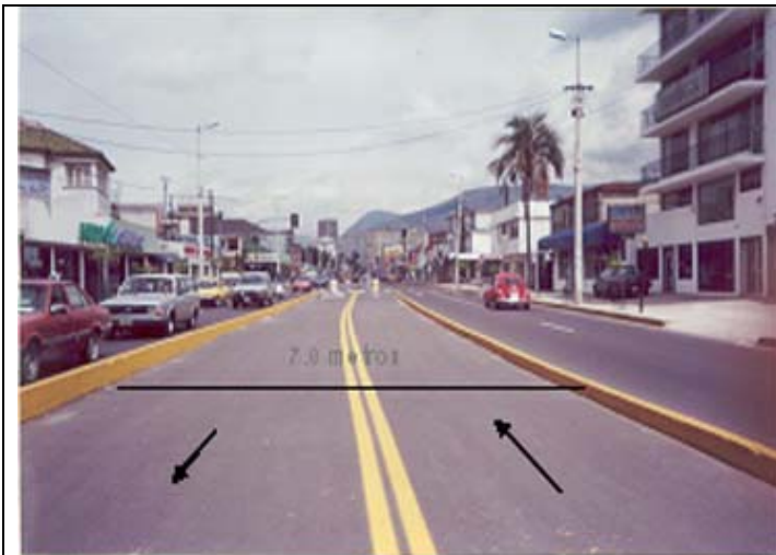
Photo 30 – Ecovía Exclusive Central Busway
