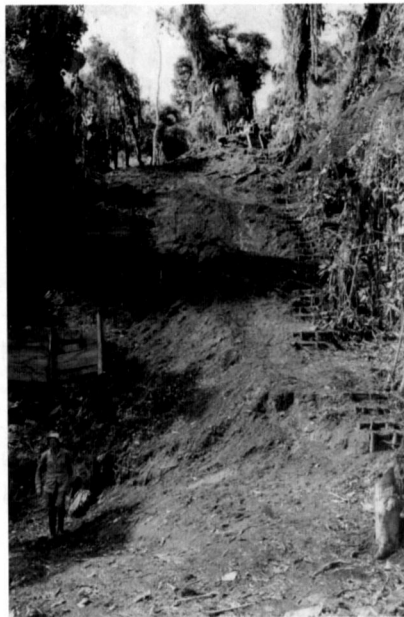
FIGURE 16: The right of way of the underground OCP pipeline varies in width from less than 7 meters in ecologically sensitive zones, such as the Andes Mountain slope in the photo, to 30 meters (Entrix, 2001). OCP passes near six active volcanoes and through seven national parks and protected areas, including a World Bank Global Environment Facility project, managed by Fundación Maquipucuan, and affects potentially an estimated 450,000 people living along its route (Entrix, 2001).
